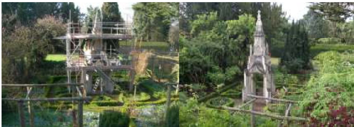
The Market Cross during restoration and after removal of scaffolding (2011)
