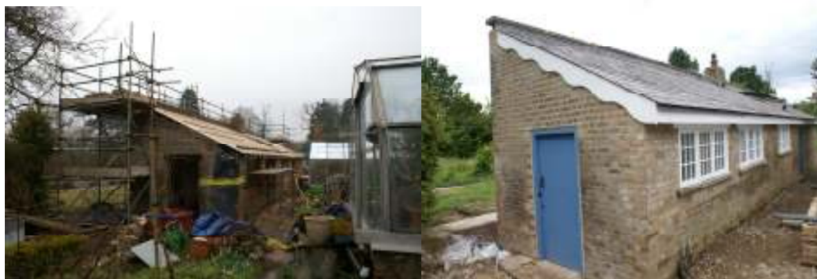
Potting Shed during and after restoration (October 2010)
