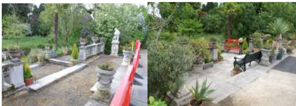
Pond Terrace during and after restoration (August 2010)
