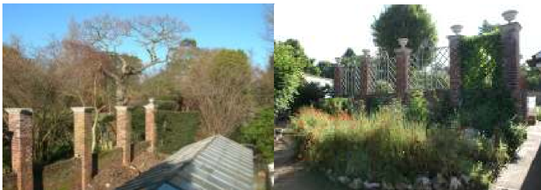
Trellis wall prior to restoration (2009) Trellis wall post restoration (2012)
