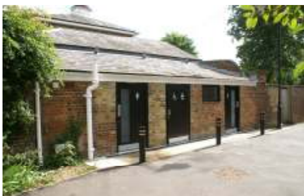
Toilet block after upgrading (2012)
