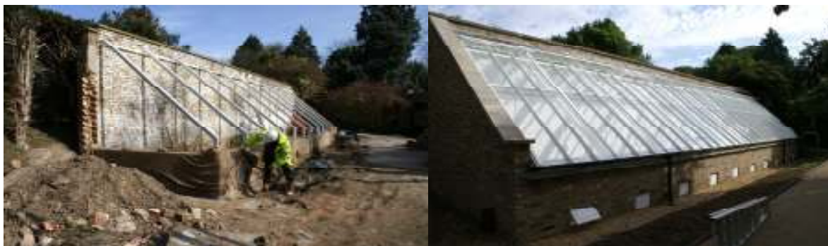
Peach House during and after restoration (October 2010)
