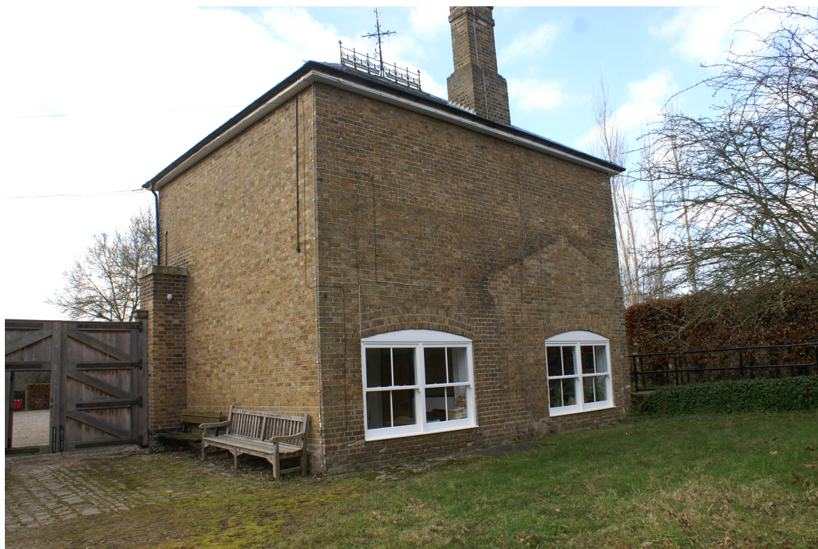
Rear of Museum with new windows 23 February 2018
