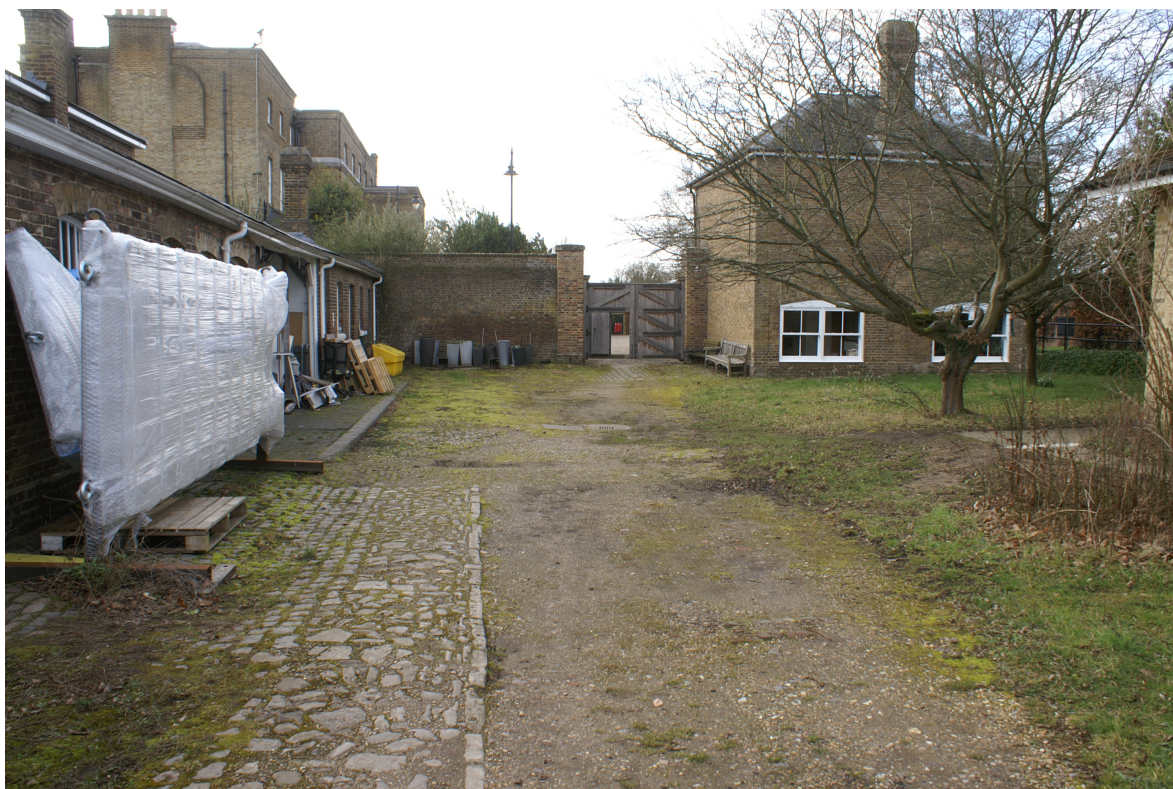
Farmyard behind Stable Block 23 February 2018
